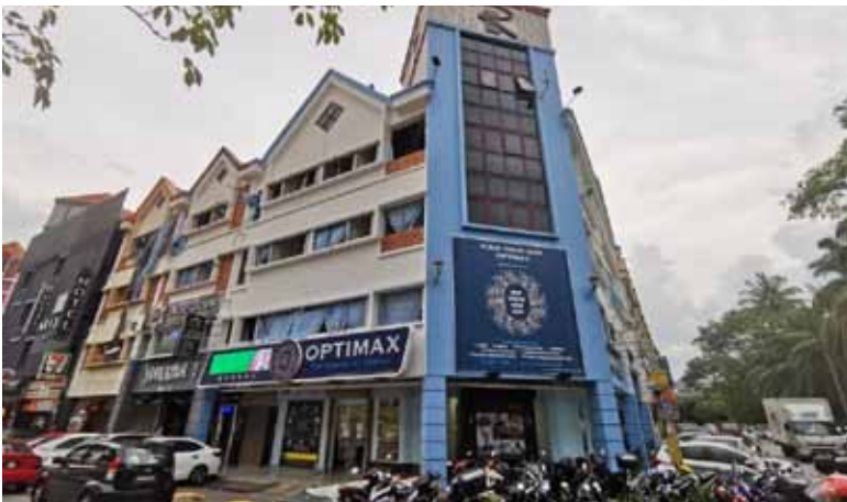
BANDAR SUNWAY - AMBULATORY CARE CENTRE
