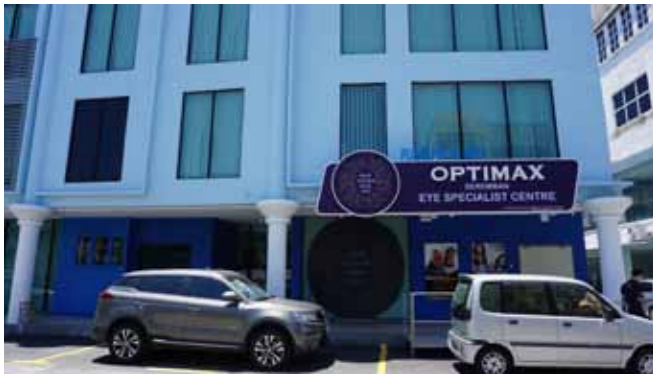
SEREMBAN - AMBULATORY CARE CENTRE
